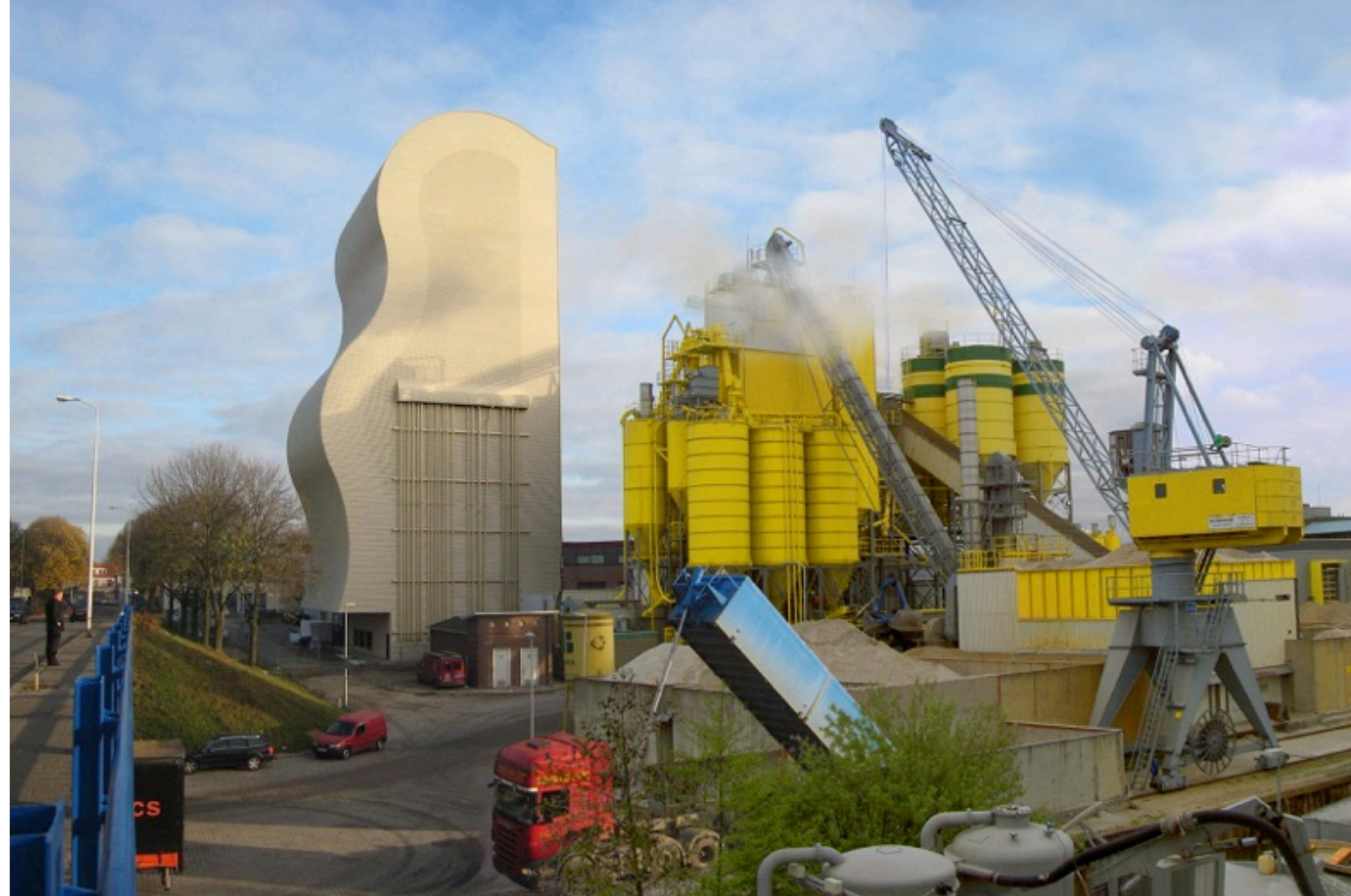
production tower for dry mortar maxima 1 saint-gobain weber beamix beatrixkade eindhoven 2009
